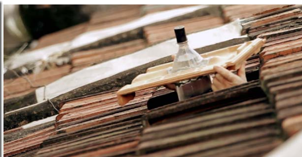
Roof tile with plastic water bottle
