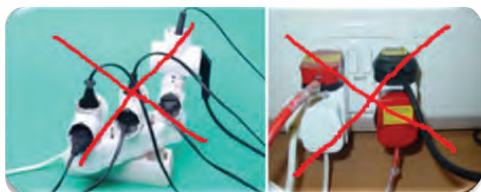
Figure 6.4. Improper use of electrical power point.
