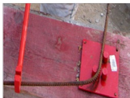
Bending of iron rod
