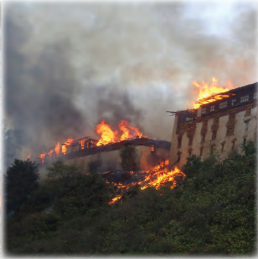
Figure 14.3(b) Building on fire
