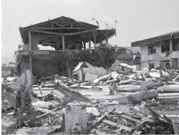
Tsunami damage in Indonesia: caused by an earthquake
