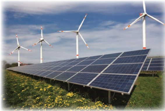
Figure 10.11 Solar panels and windmills
