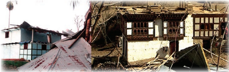
Figure 5.5. Houses affected by wind storm
