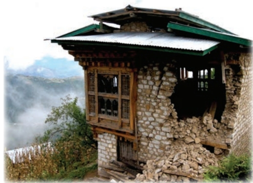
Figure 5.8 A house damaged by an earthquake
