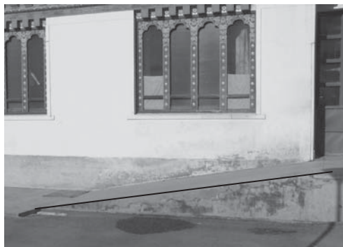
Wheelchair ramp at Paro Hospital
