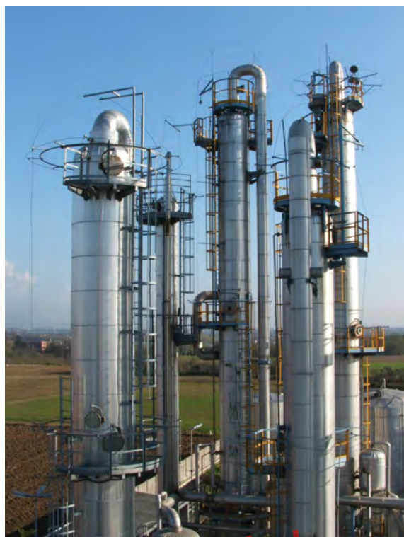
Figure 9.8 Exterior view of distillation plant.
