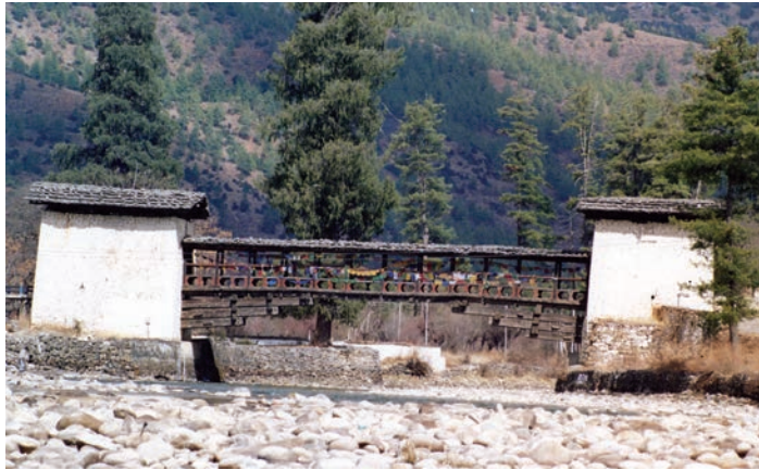
>> Figure 1.1. A cantilever bridge (Bazam རྩམ་མཉམ་)
