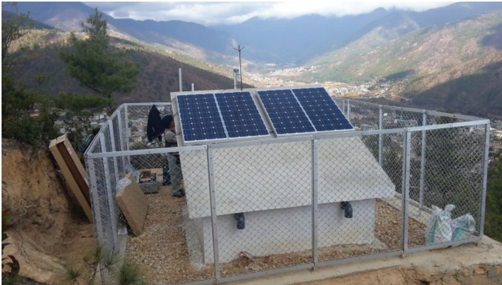
Figure 14.15: Seismic station in Thimpu. Photo: Royal Government of Bhutan
