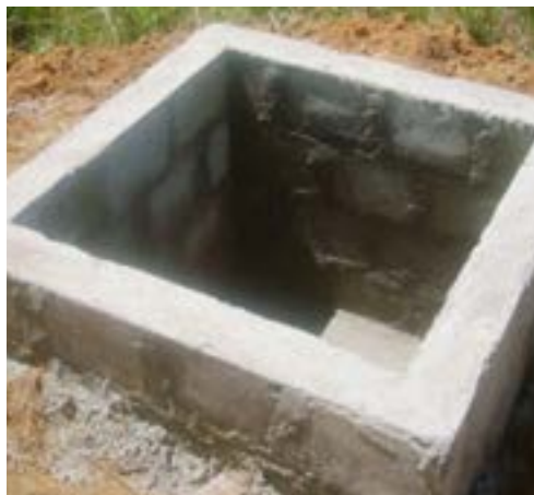
(b) Digested liquid collection unit
