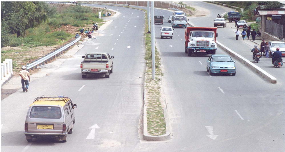
Fig. 3.1. Thimphu-Babesa Expressway(under construction)
