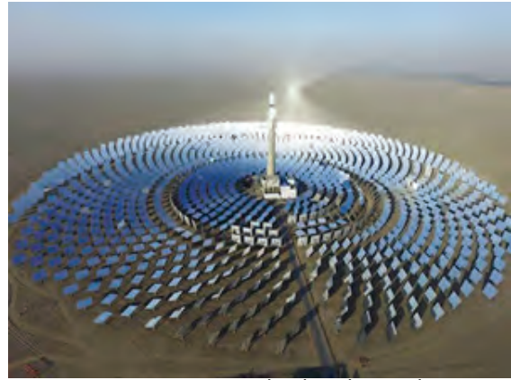
Fig. 11.2 Concentrated solar-thermal power
