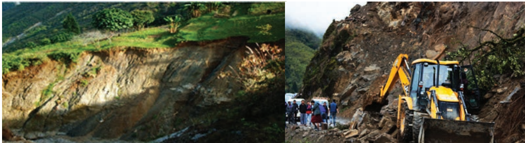
(a) Landslide encroaching agriculture field
