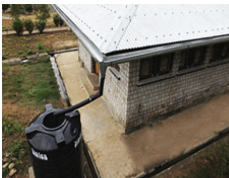
Figure 10.18. Rainwater harvest for domestic purpose
