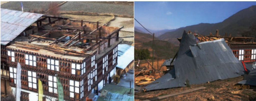
Figure 7.4. Roof torn apart by windstorm
